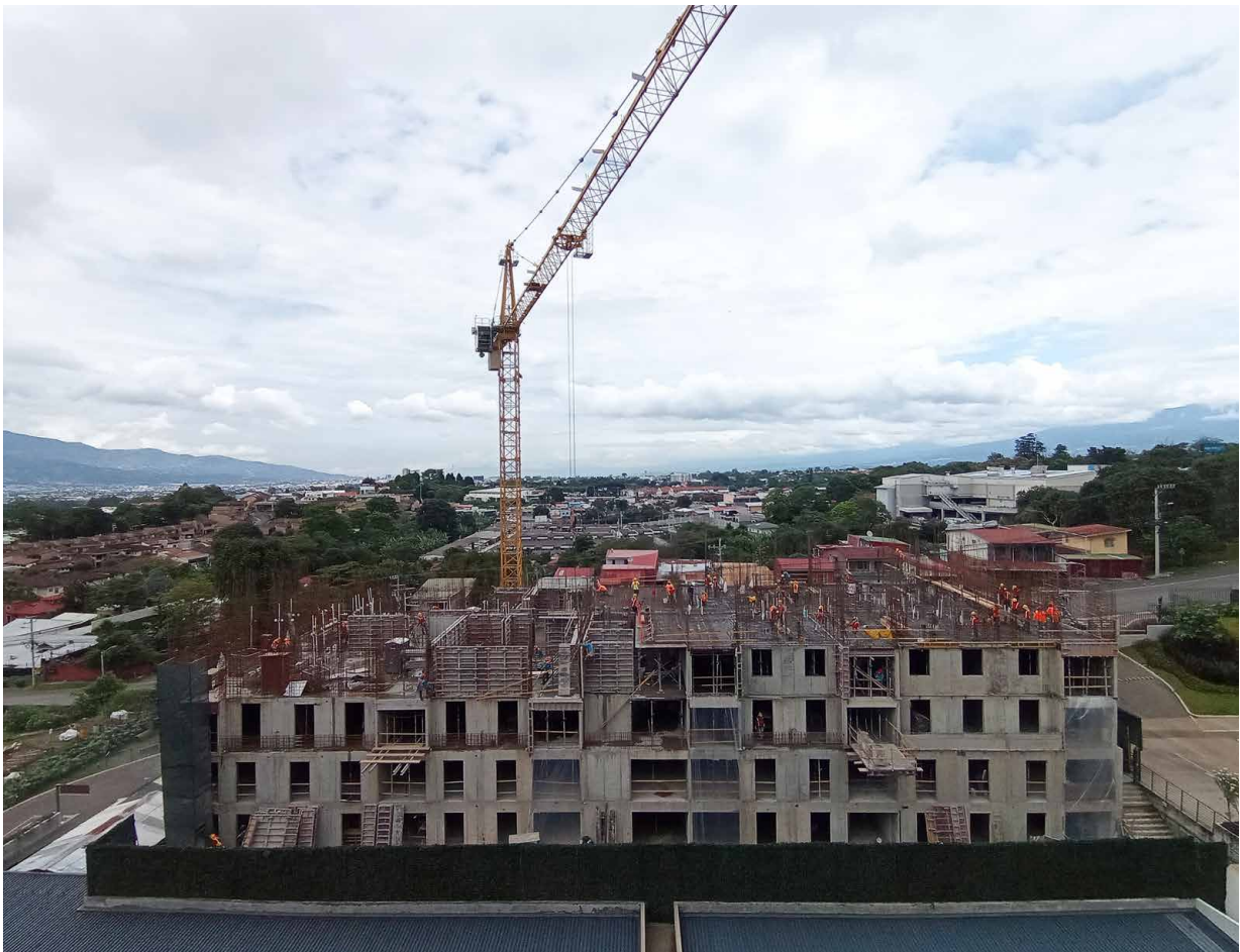
Construction of the residential tower A of Nueve84, in Aleste.
